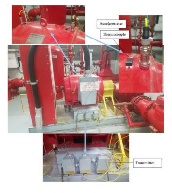
The MSMU is now being used on RHR pumps, offering safe operations for nuclear power plants and the communities they serve while creating a safer and more cost-effective work environment. INL and nuclear plants across the U.S. are working to replace the manual process for monitoring RHR pumps. They are also evaluating an expansion of the project to use vibration and contactless sensors to monitor other types of equipment in closed environments in nuclear plants.
